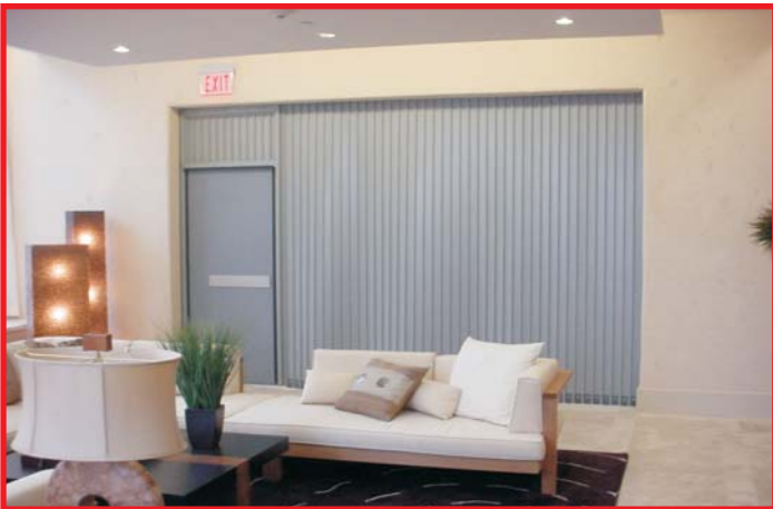
when activated the Safescape® S9000 creates both the fire & smoke protection necessary while also allowing for Egress.
